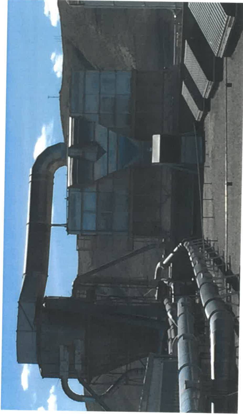
Figure 6: Facility-wide particulates air emission control equipment installed at the Permittee's building roof; cyclone (left) and baghouse (right).
