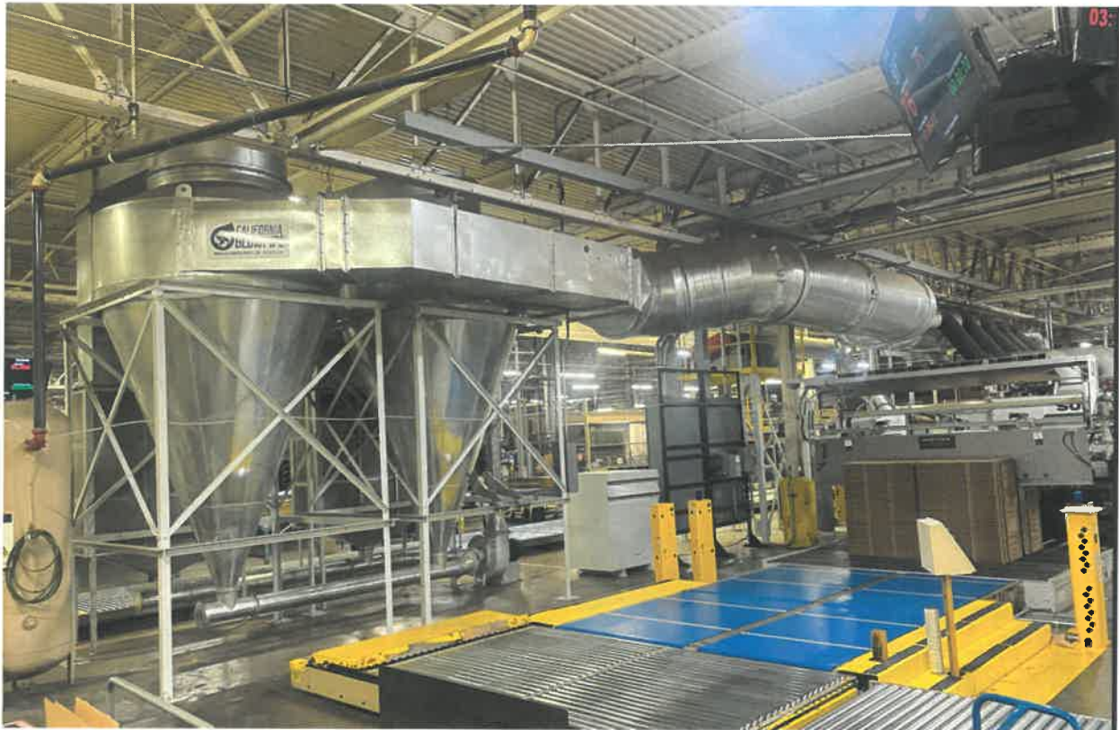
Figure 5: Flexographic portion of emissions to the Twin Handling Cyclones and after filters
