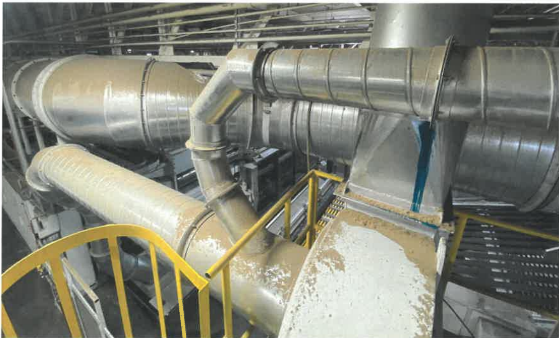
Figure 8: RDC scrap ducting connection with Twin Handling Cyclones fines exhaust to CBP #45 then to cyclone on the roof
