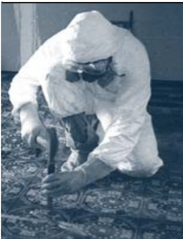
Cutting the Floor
