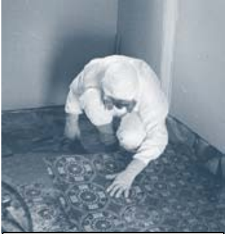
Lift and Peel up Flooring
