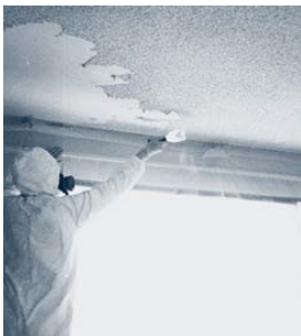
Scraping the Ceiling
