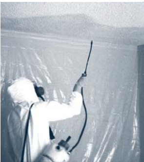
Spraying the Ceiling
