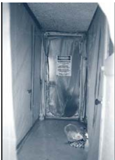
Containment Area with sign
